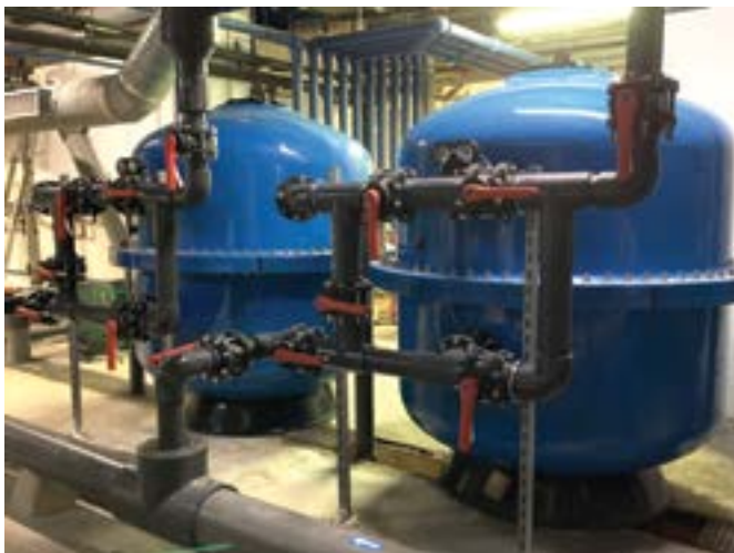
Waterco Split SMDT designed for water treatment and commercial swimming pool facilities, built using the latest in gel coated fibreglass technology and ideal for retrofitting.
